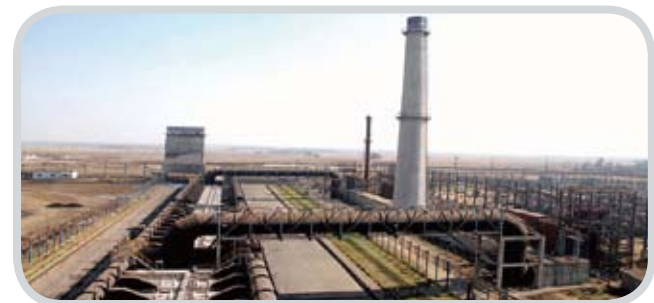
Terephthalic acid plant
