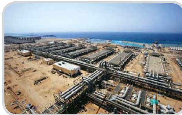
Desalination plant being constructed in Saudi Arabia by Doosan Heavy
